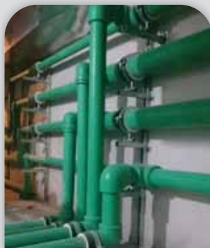
PP-RCT piping installed in an industrial process water application
