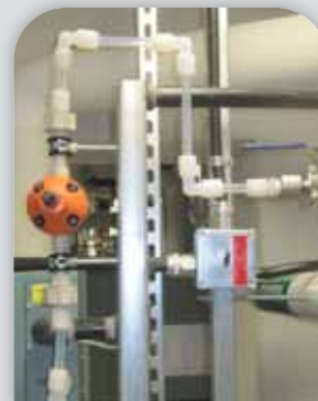
ChemFlare™ system with PFA tubing and fittings and PVDF back pressure/relief valve on medical DI water
