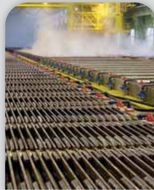
Butterfly and diaphragm valves for sulphuric acid in a copper and zinc electrowinning plant
